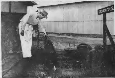
Over 2,000 samples are drawn every day. To get a true sample, the line must be flushed, but care must be used to see that no more flushing is done than necessary. If every sampler runs one quart more than is necessary to flush the line, at the end of the day 12 barrels have gone to the sewer.
